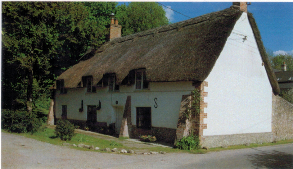
Cottages of cob at Cheselbourne, Dorset, now combined. The plinth is of flint.
