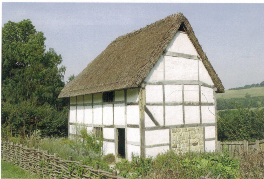
A low-status timber-framed building built for a family of simple means. (Poplar Cottage, Weald & Downland Open Air Museum.)
